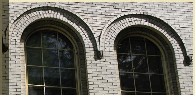
The thin sash above the arched windows extends to the base of the next window to rest on a shield shaped cul-de-lampe.
